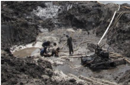
Typical on-shore TI unit
