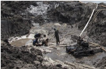
Typical on-shore TI unit
