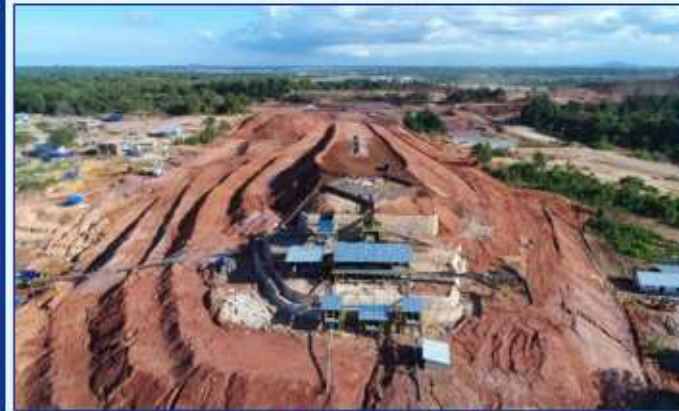
Mineral Processing Plant Expertise in Managing of Mineral Processing Operation
